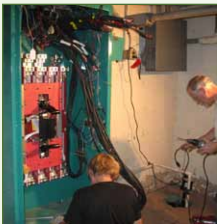
Work to improve generator operations at Town Hall
