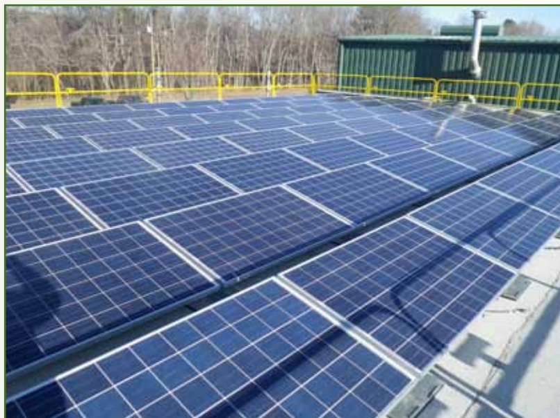
Solar panel installation on highway garage roof
