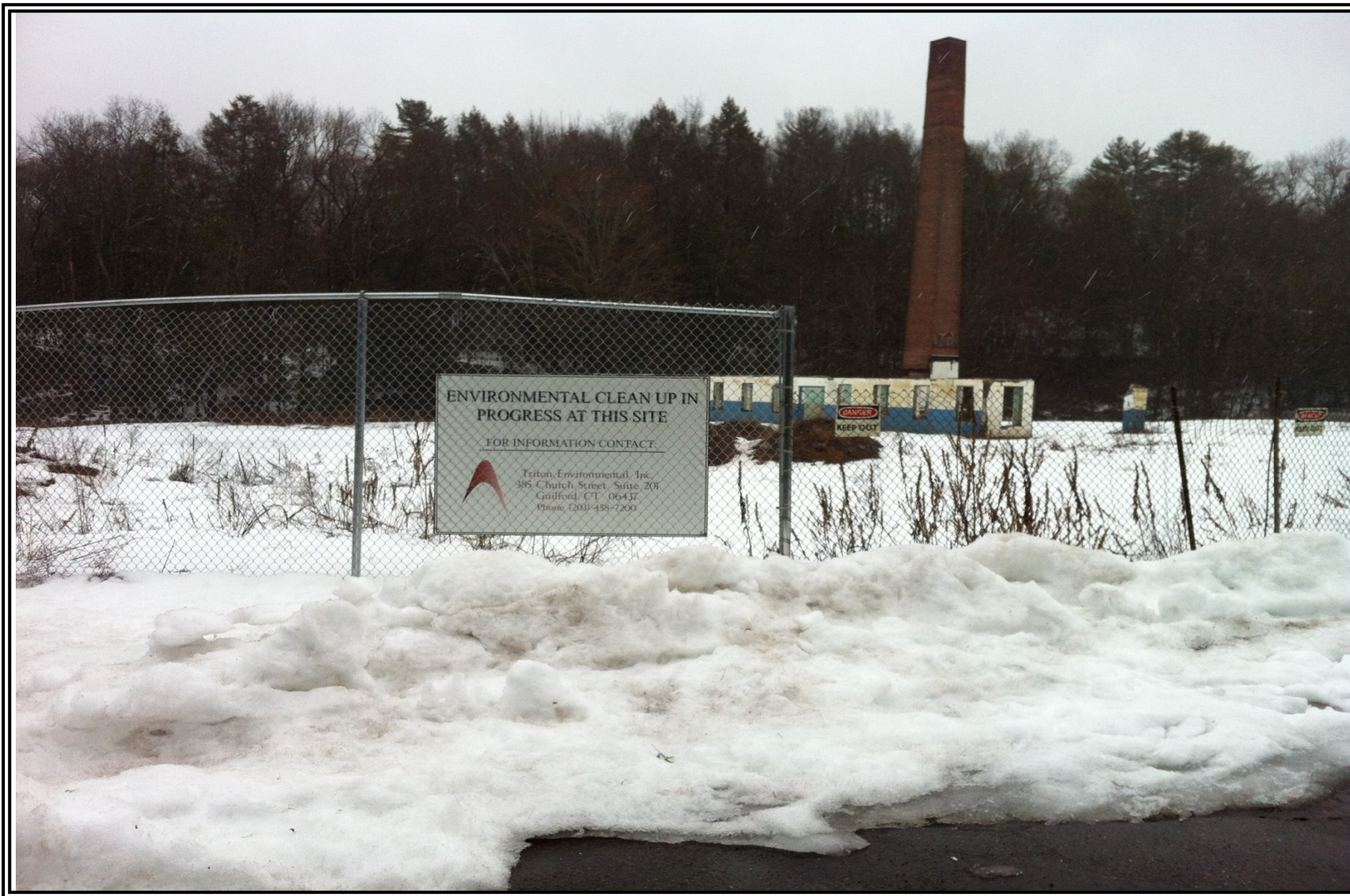
Public Notice Sign Installed by Triton Environmental, Inc. on February 27, 2013
