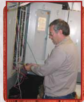
Facilities staff members fine-tune air conditioning system to ensure optimum performance.
