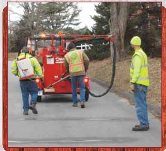
Town Highway Division staff sealing road cracks.
