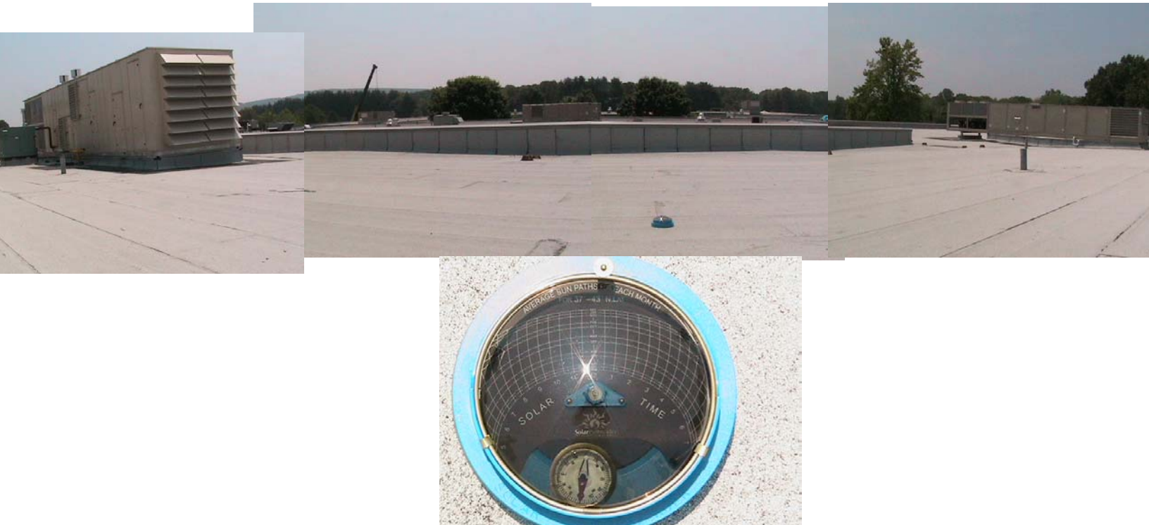
Fig 20: Panoramic View and Pathfinder of optimal array location on “A” Wing
