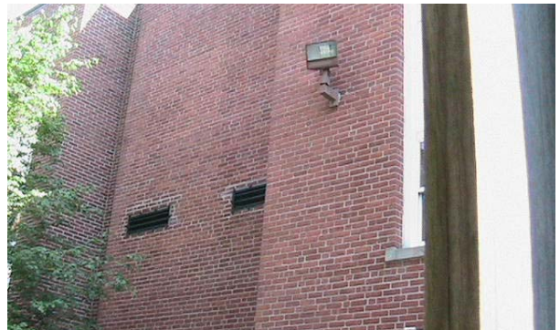
Fig 5: View of generator conduit into building and of west side wall.
