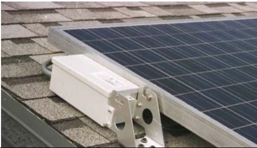
Fig 14: Example of Roof Jack system for standard modules mounted on slant roof
