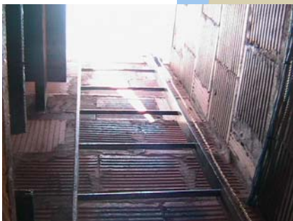
Fig 2: Roof Hatch at Glastonbury Town Hall
