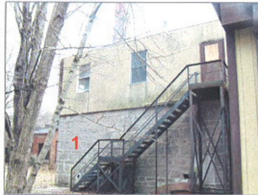
East and north sides of Building 1 (granite walls of Main Mill, 1836, remain). Upper section has been rebuilt.
