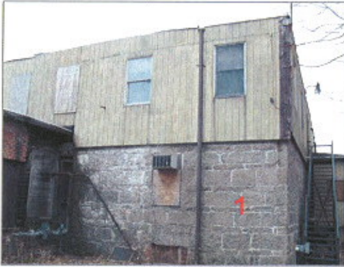
East and north sides of Building 1 (granite walls of Main Mill, 1836, remain). Upper section has been rebuilt.
