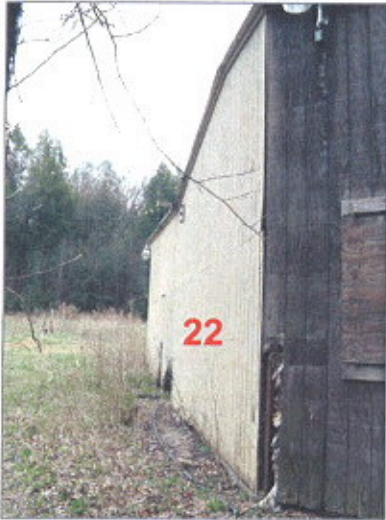
East side of Building 22 (1983).
