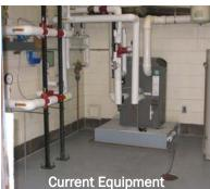
Equipment bay retrofitted with two vacuum-exhausted radiant heaters; new high-efficiency condensing boiler occupies less than one-fourth space of previous boiler
