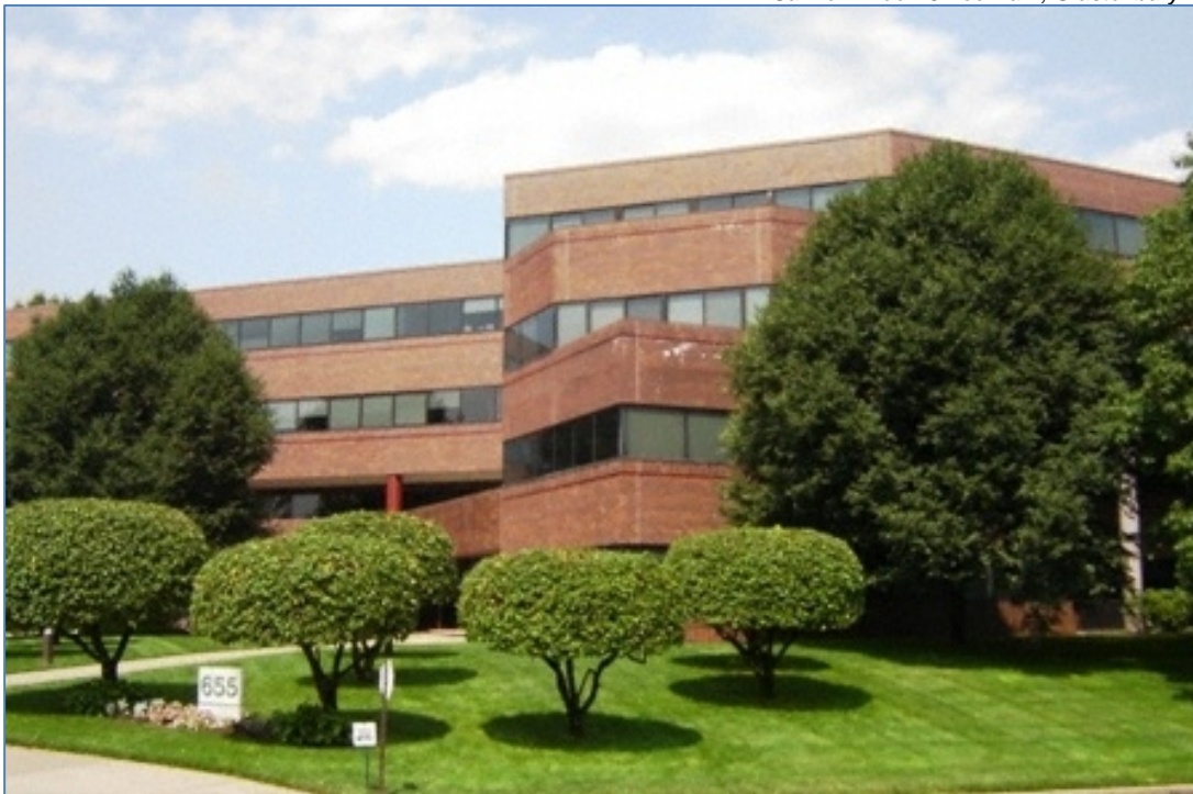
Salmon Brook Office Park, Glastonbury
