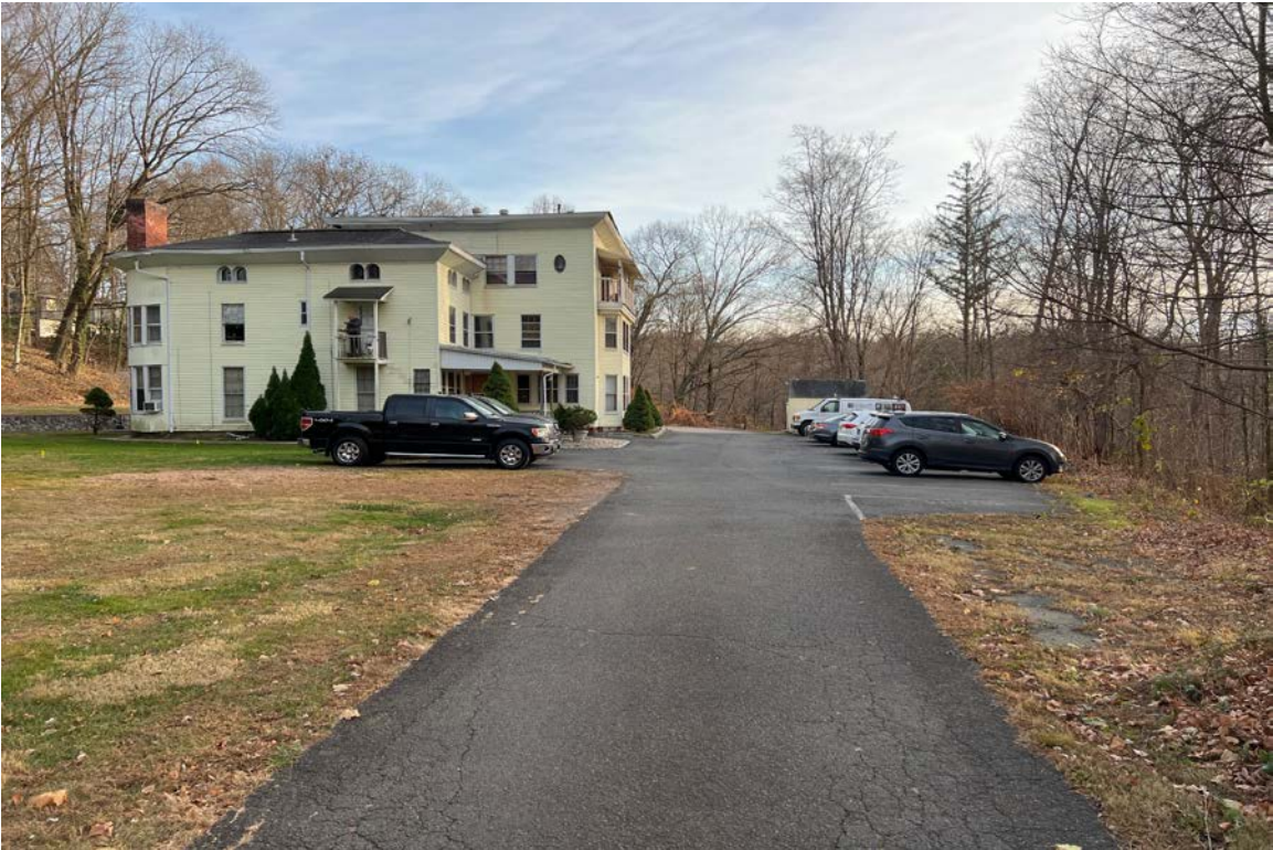
Photo 1: View of existing 6-unit multi-family building looking south. A portion of the western parking lot, the shed at the far end of the parking lot, and cleared/graded slope encroach into the 100-foot upland review area.
