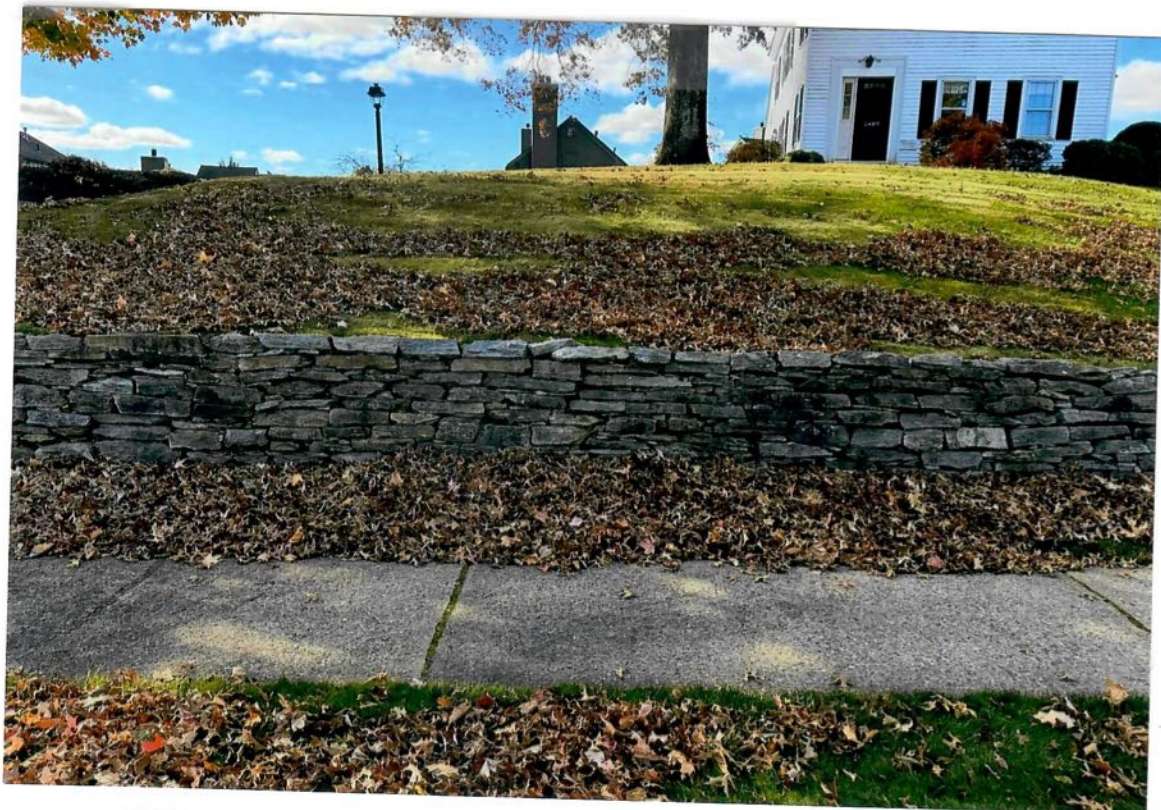
SITE RETAINING WALL ALONG MAIN STREET
