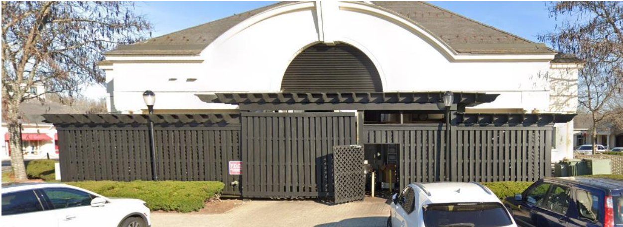
Figure 2 Black wooden enclosure adjacent to the building. New black fence will apport a more cohesive image at The Shops at Somerset Square
