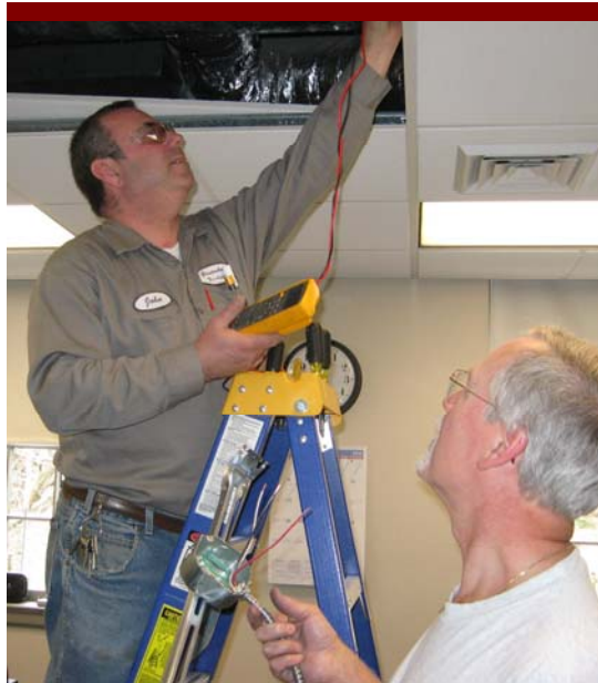
Town Facilities crew working on ceiling system during recent renovation.
