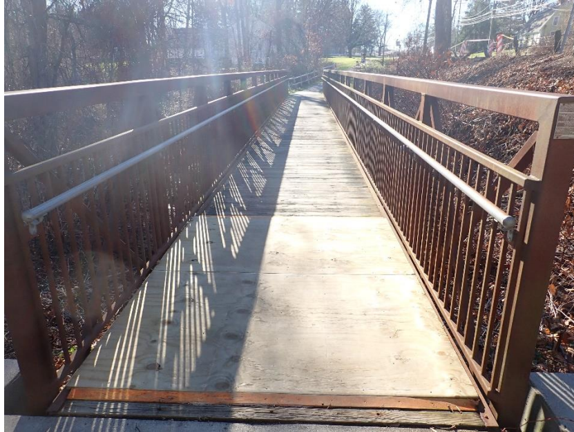
View of Bridge from North approach
