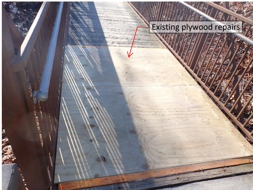
North end of bridge
