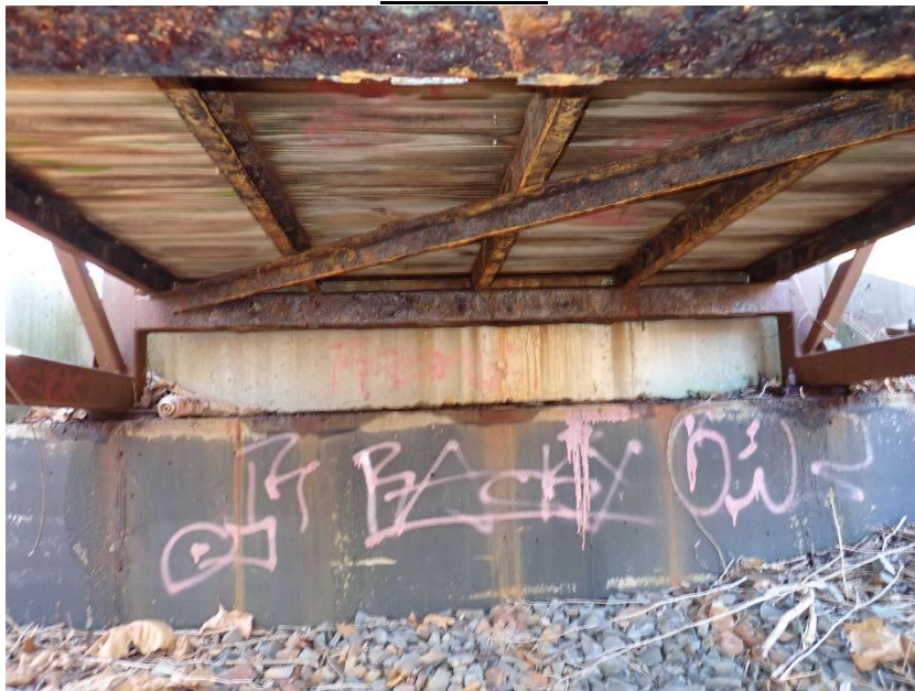
North Abutment (Looking North)
