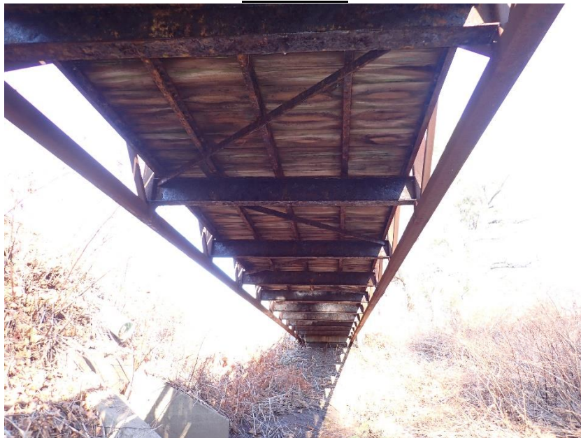
Typical underside of the bridge
