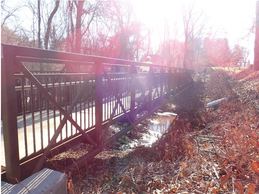
West Elevation (Downstream)
