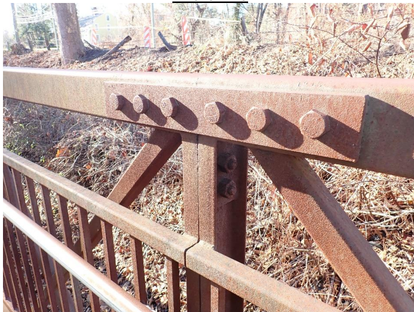
Splice joint at mid-span of bridge
