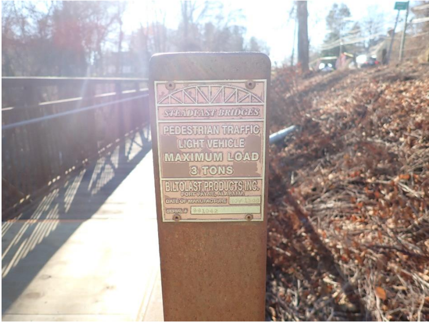
Bridge Id Plate Northwest end
