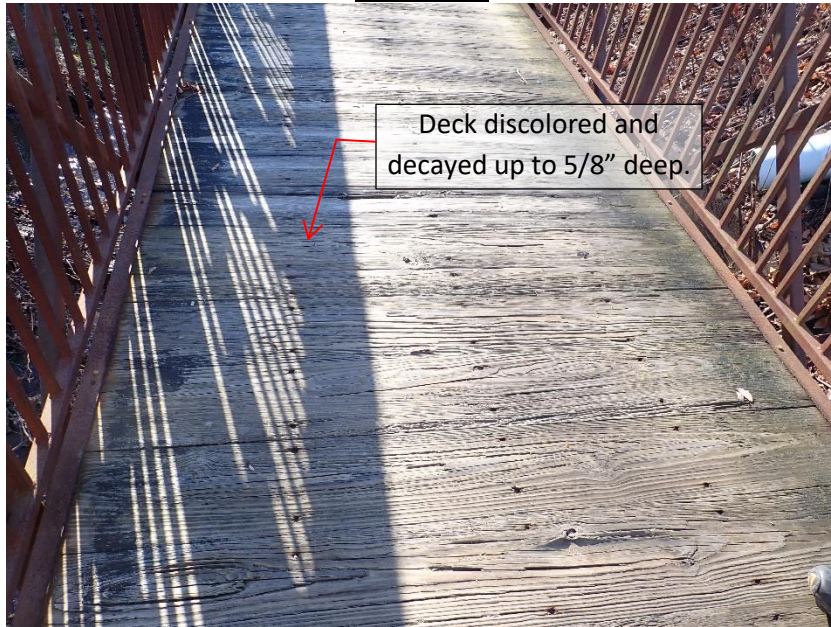
Typical top of bridge deck
