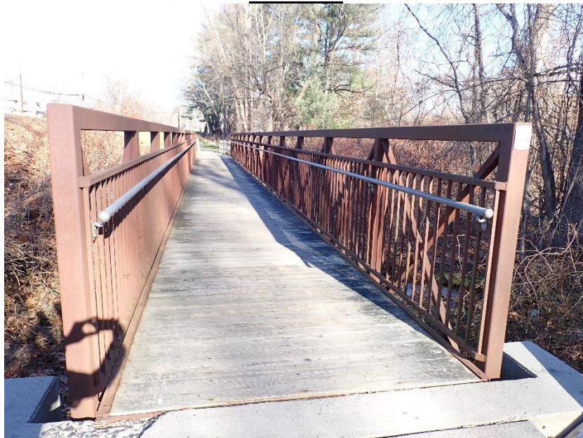
View of Bridge from South approach
