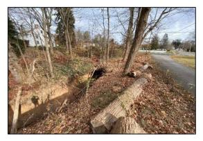
an as-needed basis as determined by the Town Manager. Recent issues have been encountered with discovery of badly deteriorated metal drainage pipe installations. Additionally, the increasing frequency of intense precipitation events has revealed system capacity issues which may require modification to prevent flood related private property damage.
