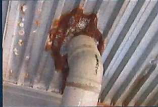
Corrosion at Scupper Penetration
