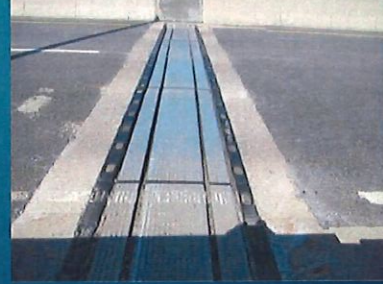
Modular Joint at ends of Main Span Unit
