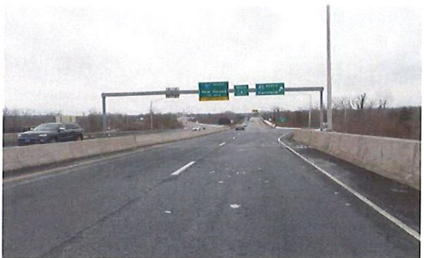
Bridge From The West Approach, Northbound Lane Shown
