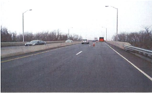
Bridge From The East Approach, Southbound Lane Shown
