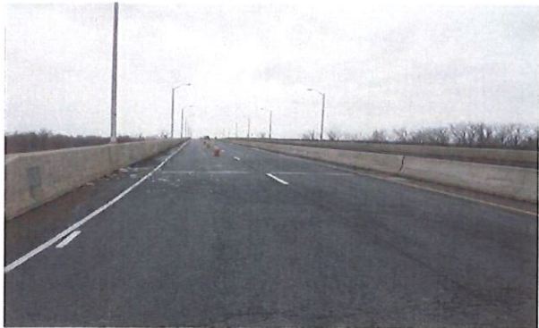
Bridge From The West Approach, Southbound Lane Shown
