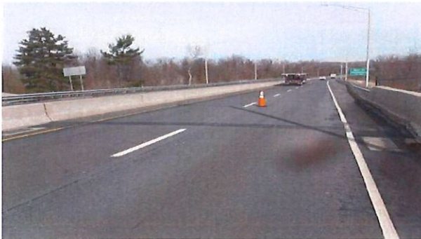
Bridge From The east Approach, Northbound Lane Shown
