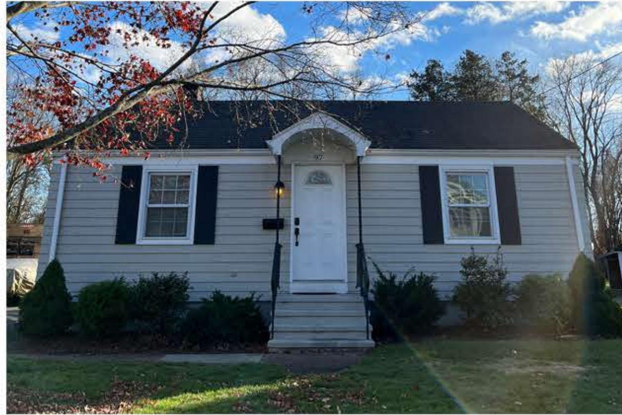
EXISTING SOUTH SIDE
