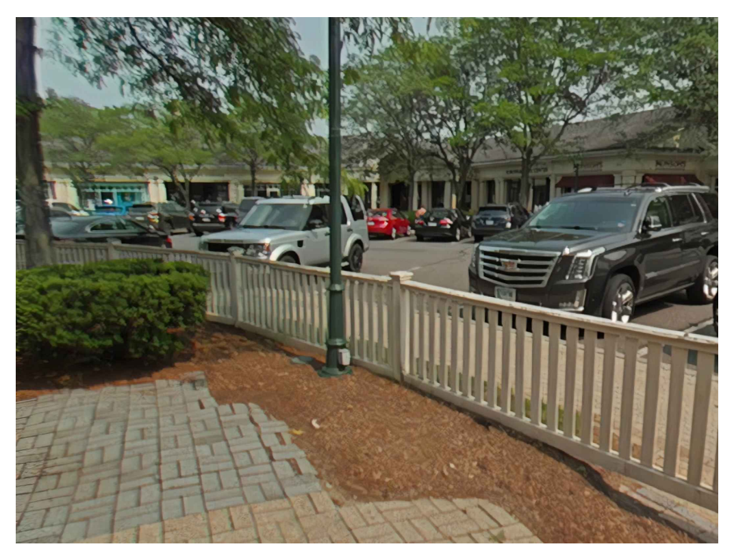
EXISTING FENCE TO REMAIN GC TO CLEAN, REPAIR AND REPAINT AS NEEDED
