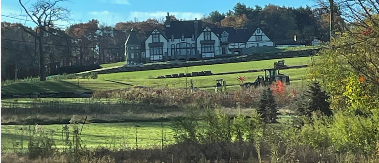
Photo taken by S. Simone, October 31, 2023: Machine work being conducted near the pond and watercourse as viewed from Matson Hill Rd.
