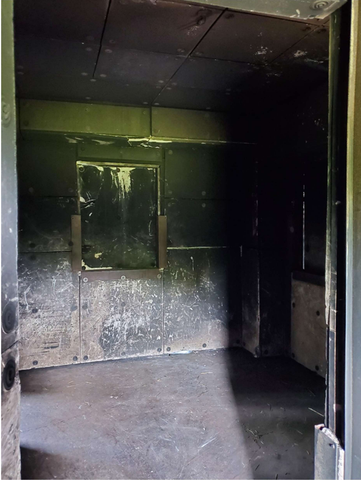
Existing Second Floor Burn Room – Tile Replacement
