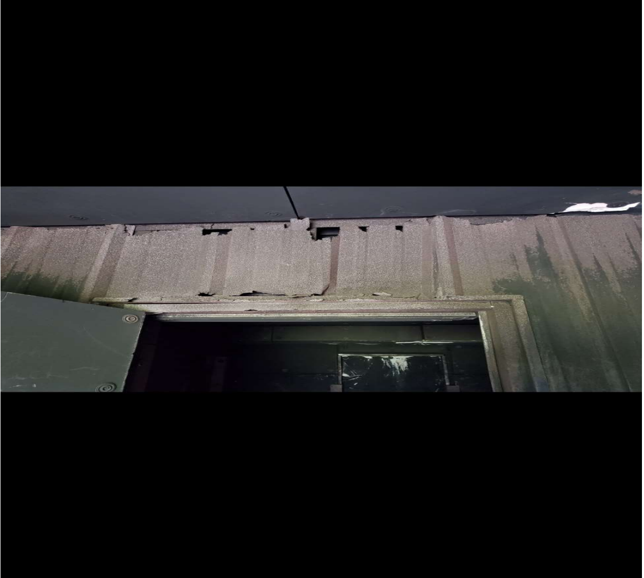
Existing Second Floor Burn Room Door Frame and Wall Replacement
