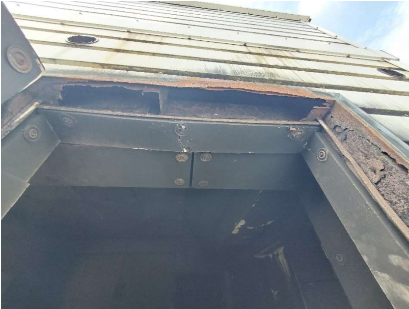
Existing Second Floor “B” Side Burn Room Window – Frame Replacement
