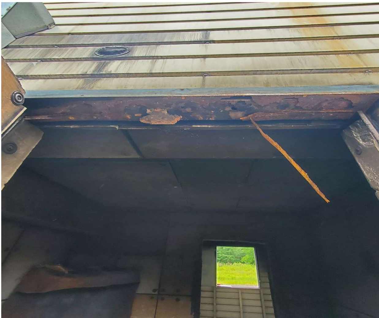
First Floor Burn Room "A" side window frame replacement
