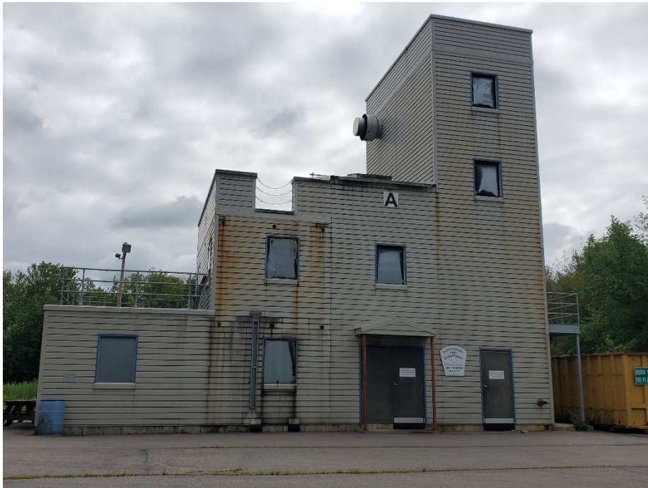
Glastonbury Fire Department – Fire Training Facility
