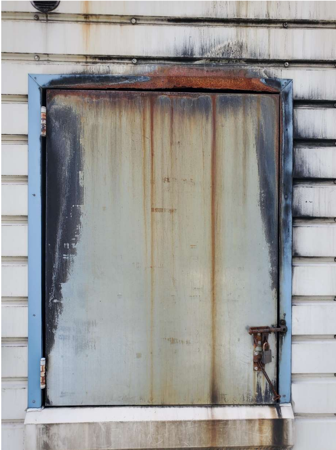
Existing Second Floor “B” Side Burn Room Window – Frame Replacement
