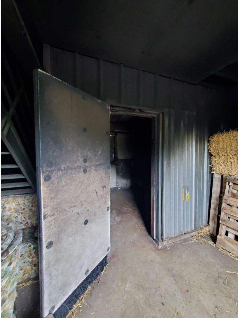
Existing First Floor Burn Room
