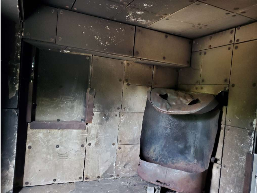
Existing Second Floor Burn Room – Tile Replacement
