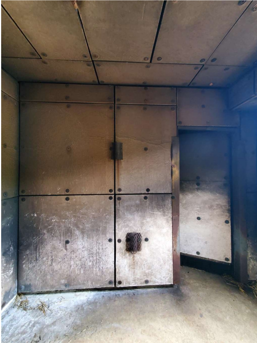
Existing First Floor Burn Room – Tile replacement / upgrade
