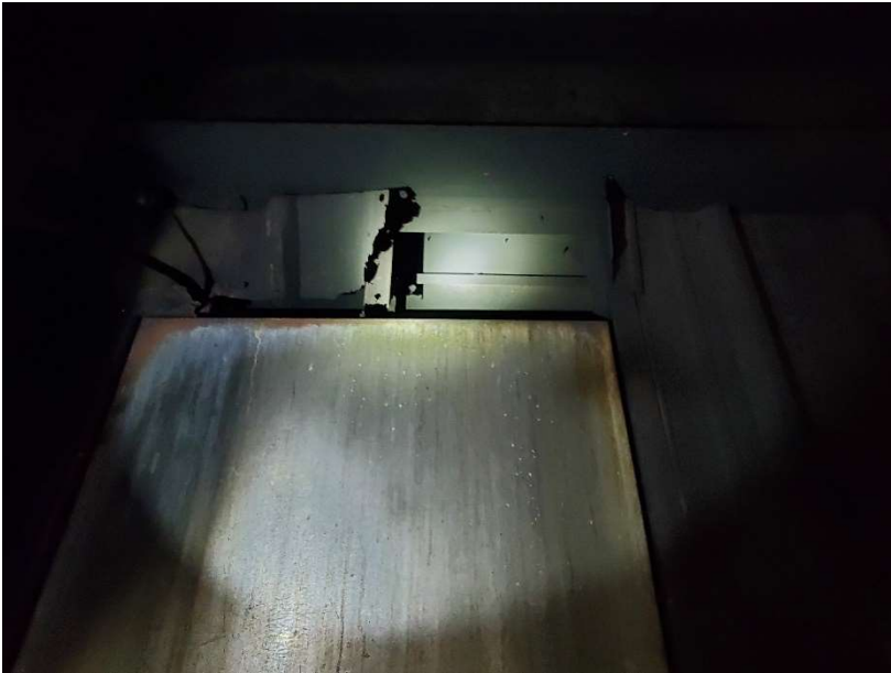
Room – Entry Door Frame / Wall Replacement
