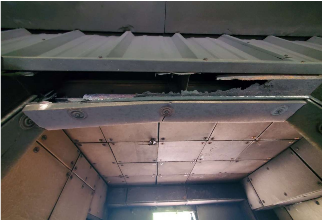
Existing First Floor Burn Room – Entry Door Frame Replacement
