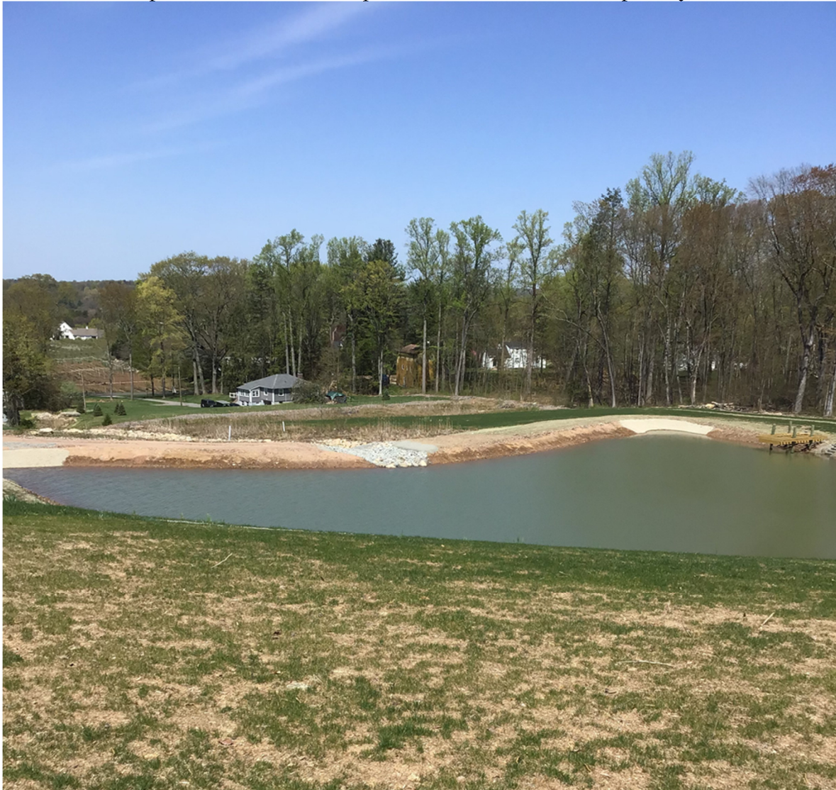
Photo 1 taken April 21, 2023: View of pond and established stone spillway.
