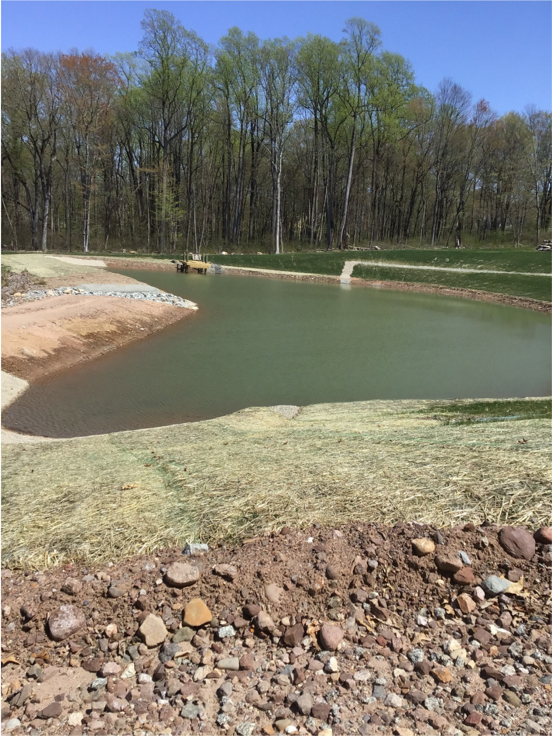
Photo 2 taken April 21, 2023: Profile view of pond and established stone spillway.
