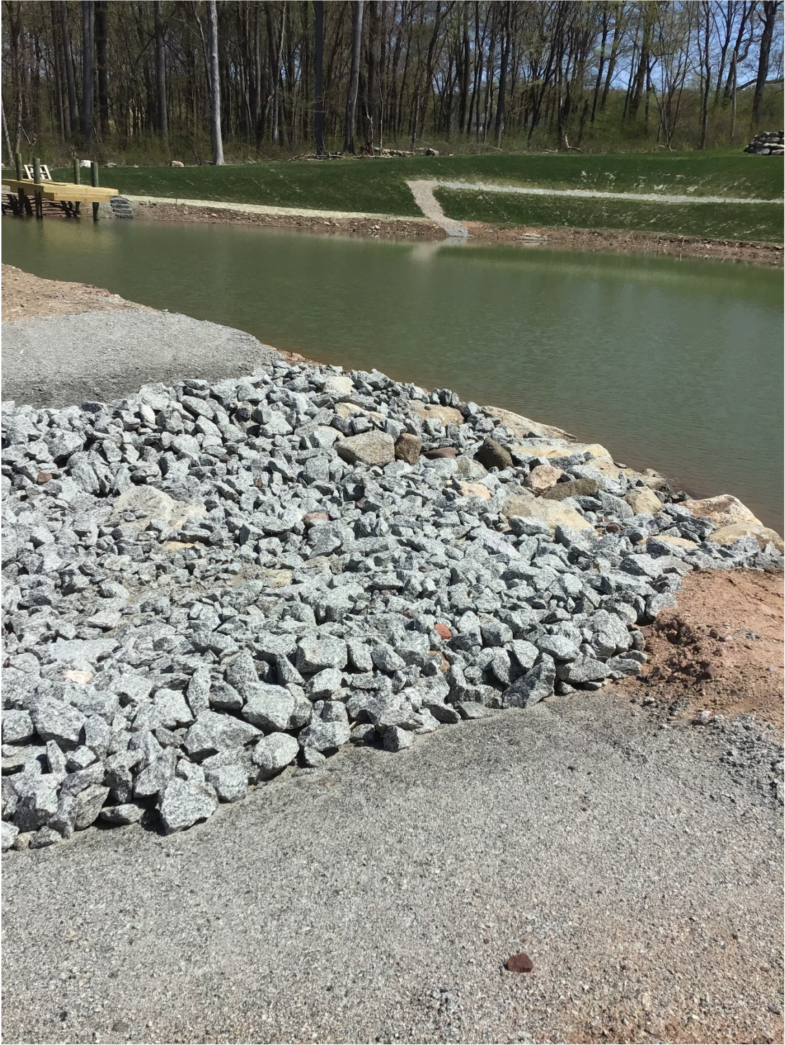
Photo 3 taken April 21, 2023: Existing spillway with stabilized stone.
