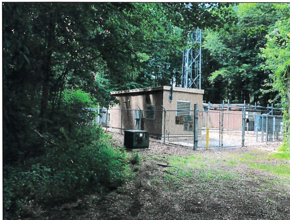
Photo 6: cell tower facility. Looking northwest
