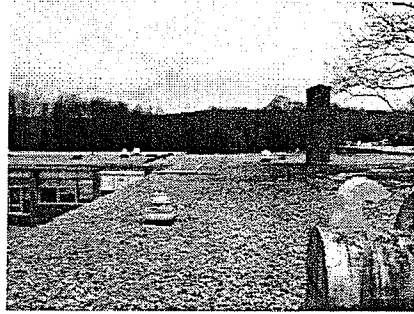
Overview of ballasted EPDM (P4090541)
