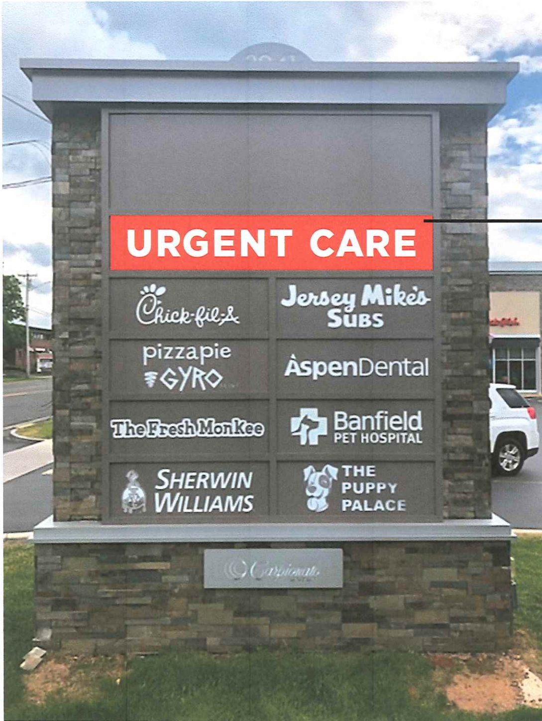
Aluminum face with cut-out text backed up with white acrylic
