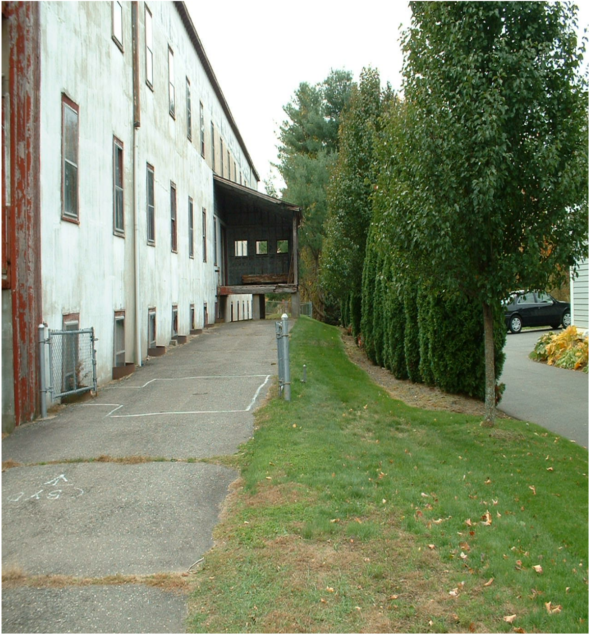
Looking south along the western (right) side of the property.
