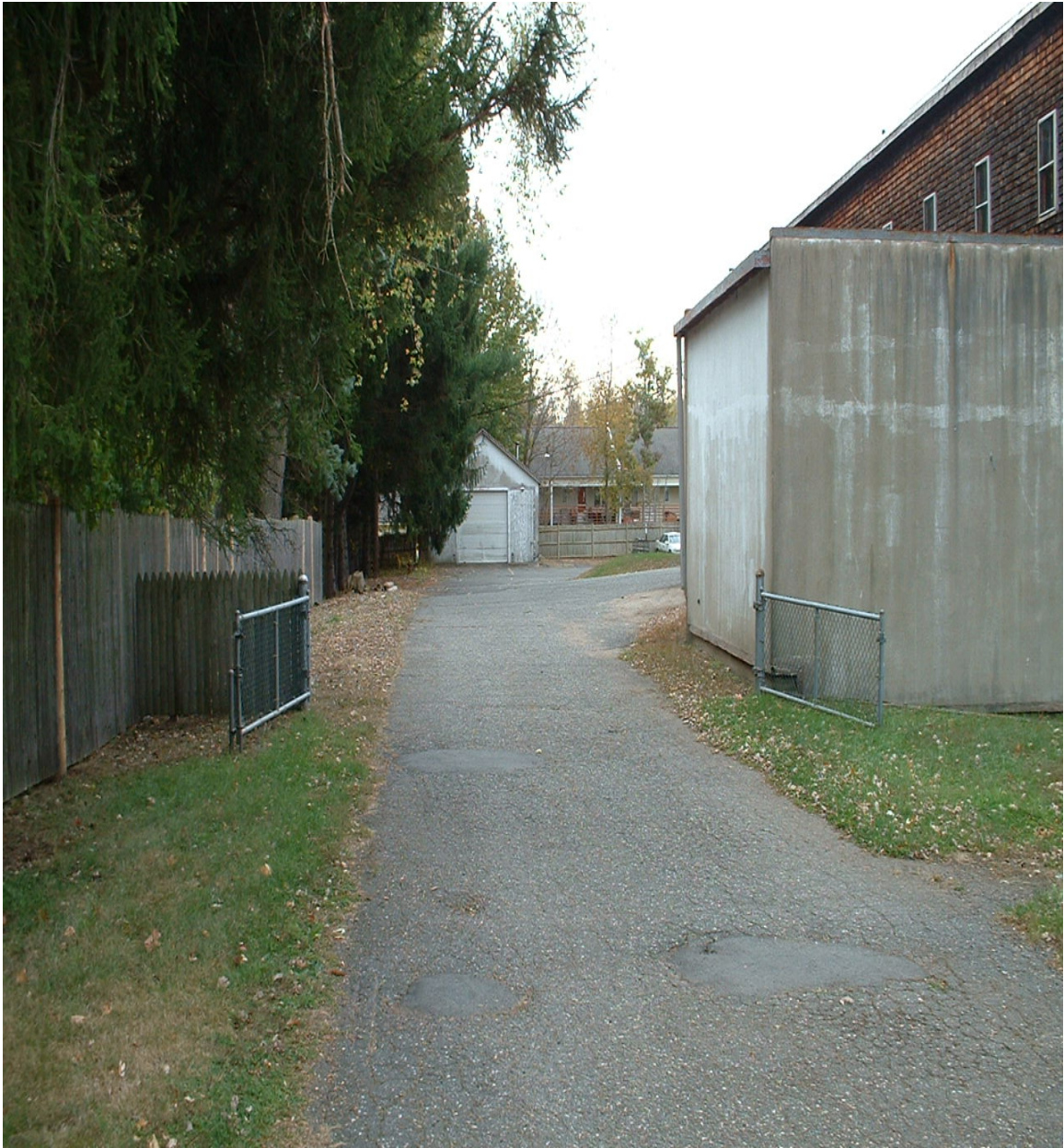
Looking south along the left (eastern) side of the site.
