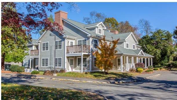
Rosenthal Gardens in Branford – 17-unit low-income senior housing in a converted historic home and new construction (NeighborWorks New Horizons)
