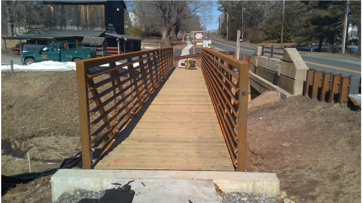
Main St Sidewalk corridor during construction.
