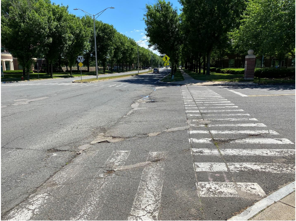
Pedestrian Crossing prior to construction
