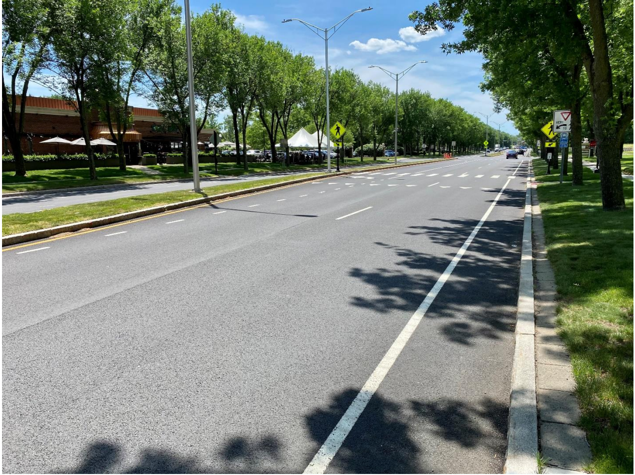
Wider shoulder width to accommodate cyclists post construction
