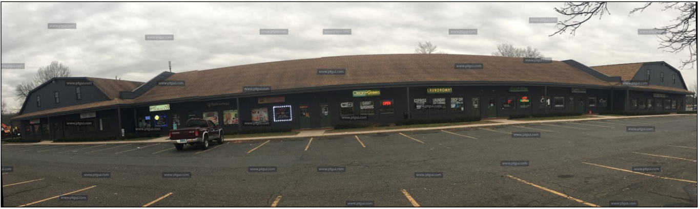
View from parking lot of 3039 Main Street looking south
