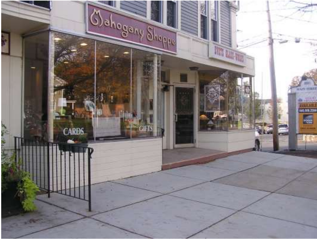
Active store fronts of 2283-2289 Main Street. Upper floor appeared vacant (October 2021).
