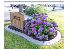
Example of an appropriately shielded utility structure
