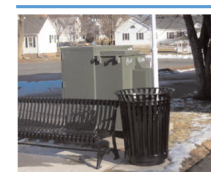
Example of an exposed utility structure which is not encouraged
