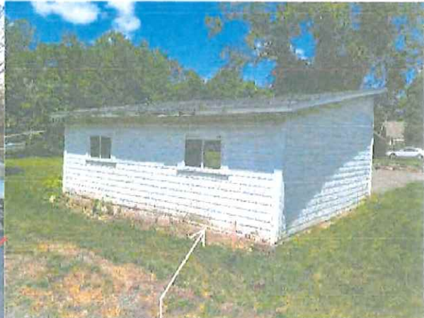
Loose Single Course of CMU to be removed
