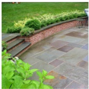
BRICK-FACED SEAT WALL WITH STONE CAP
