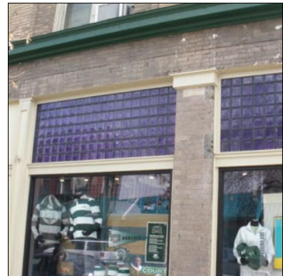
Glass block in transom of storefront
