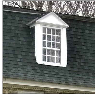
Dormer in asphalt shingle roof
