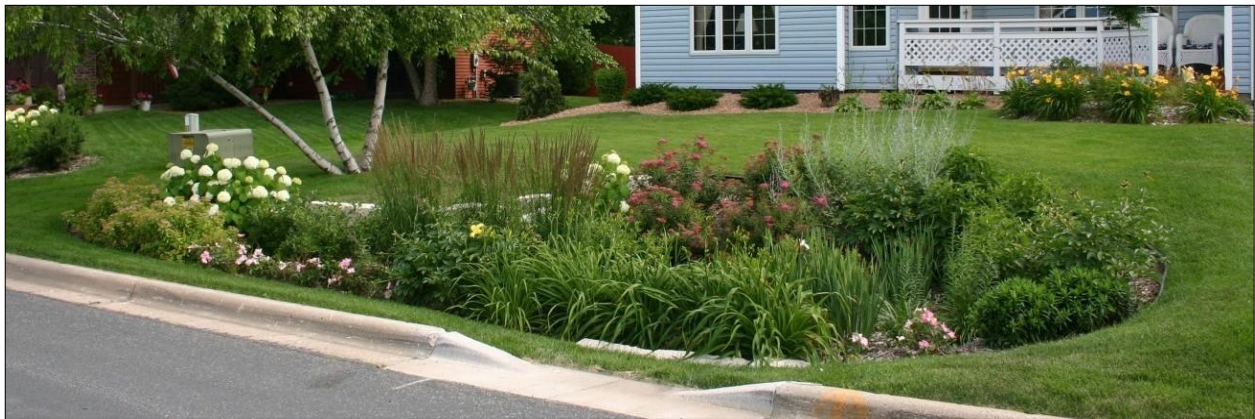
Rain garden for stormwater infiltration
