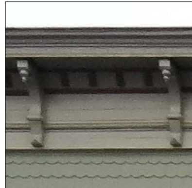
Projecting cornice at parapet
