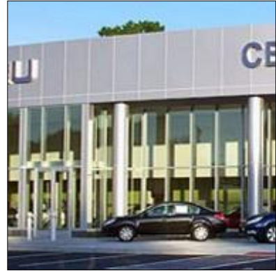
Glass curtainwall system
