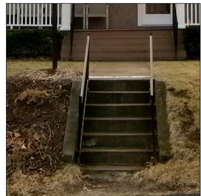
Planted embankment and grade change
