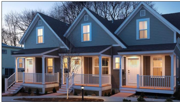
Attached single family cottages
