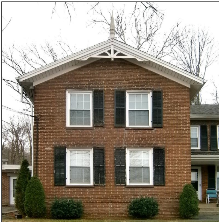
Eaves – projecting from the gable end of the building form – with decorative trim
