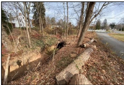
Department: Physical Services Project Title: General Storm Drainage Improvements
