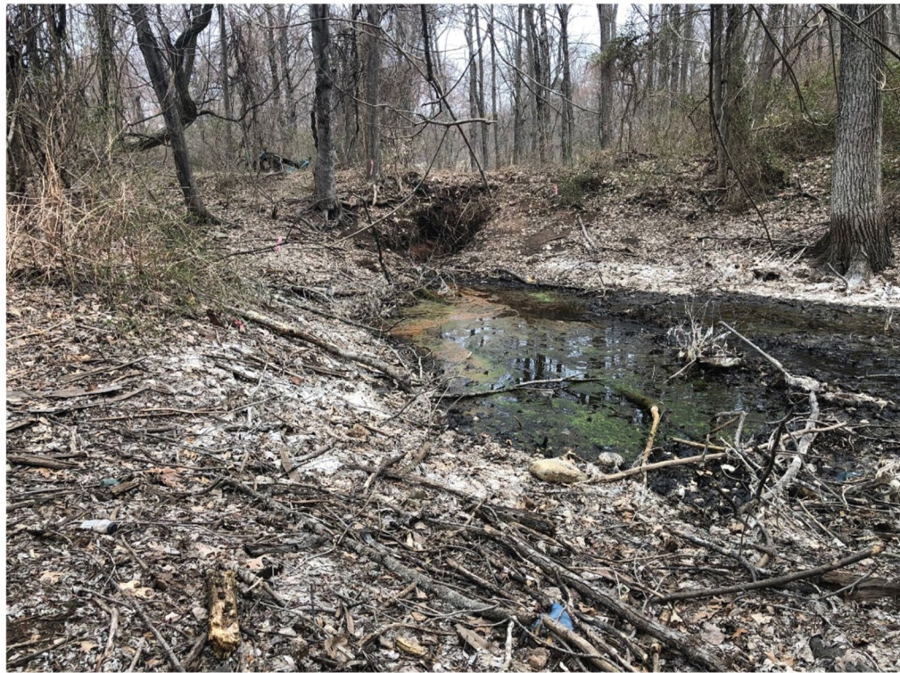
Photo 4: view of northeast corner of wetland showing where the vernal pool outlets into the culvert. Note iron staining near culvert inlet.
