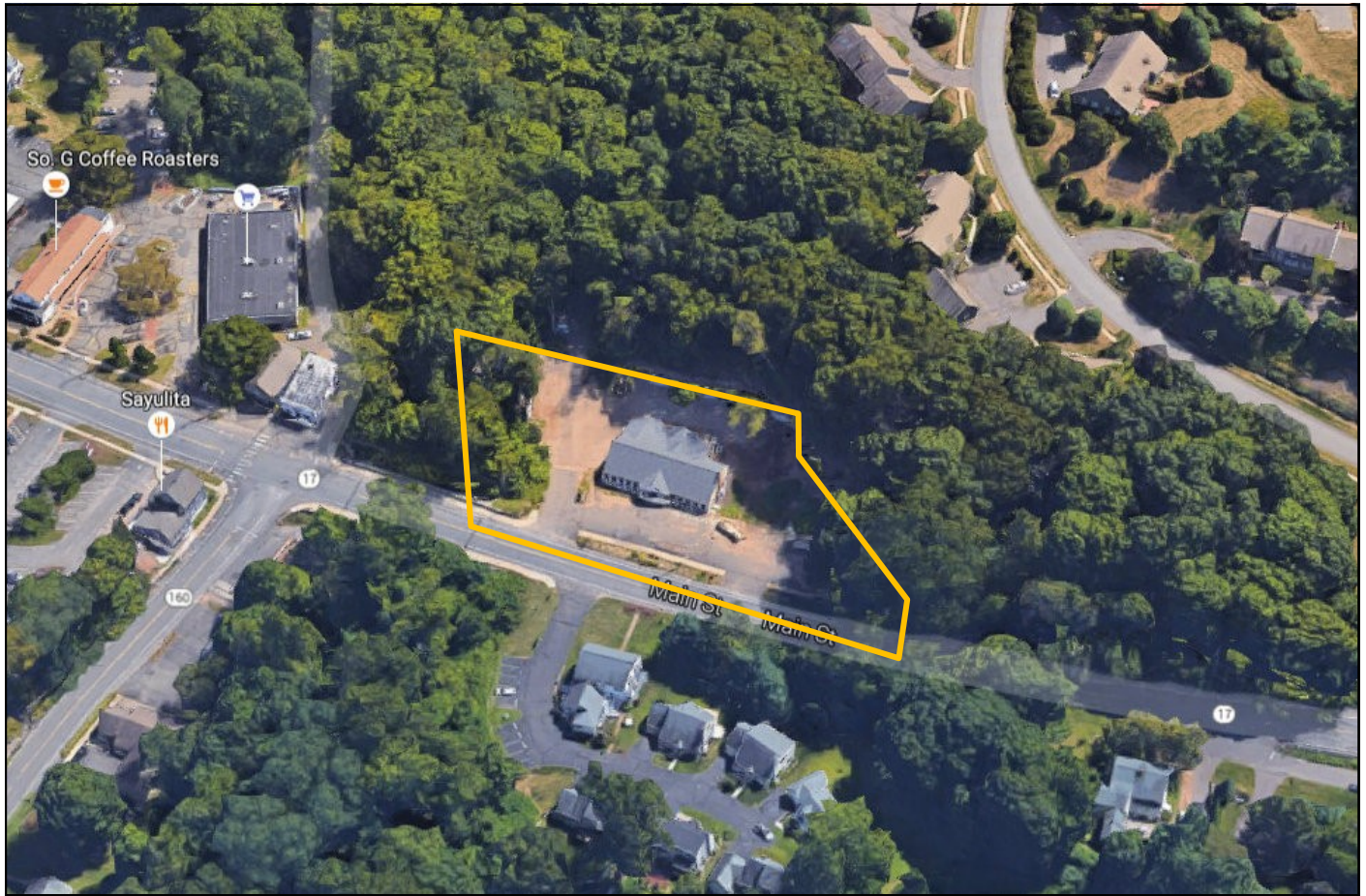
Aerial view of 840 Main Street looking east
