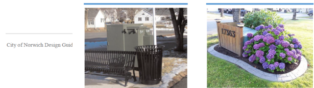
City of Norwich Design Guid Example of an exposed utility structure which is not encouraged Example of an appropriately shielded utility structure
