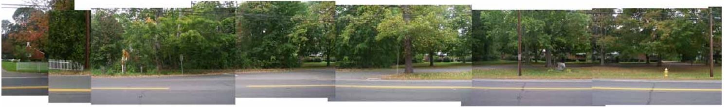
Post Road West (North Elevation):
