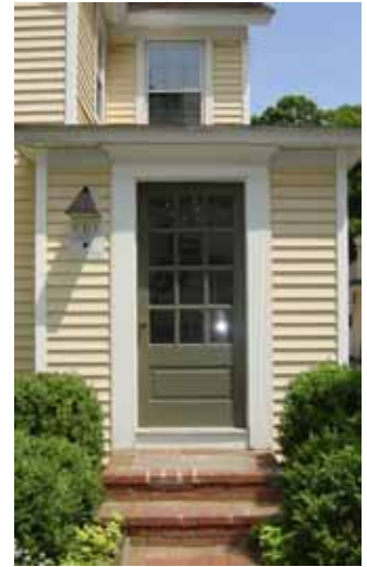
This door has an appropriate frame and real muntins.
