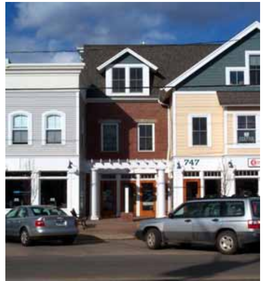
A combination of the preferred window styles can create interesting storefront compositions.
