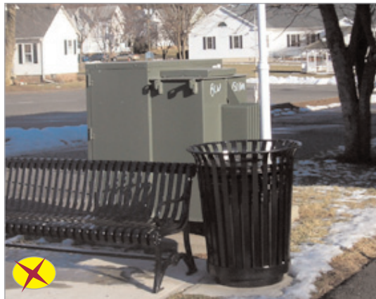
Benches and trash receptacles do not sufficiently screen utilities. Utility should be out of sight, or view.
