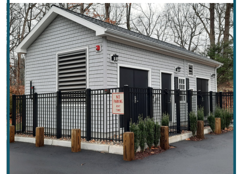
Cider Mill Pump Station
