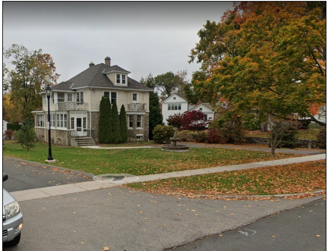
Street view of 2157 Main Street looking northwest
