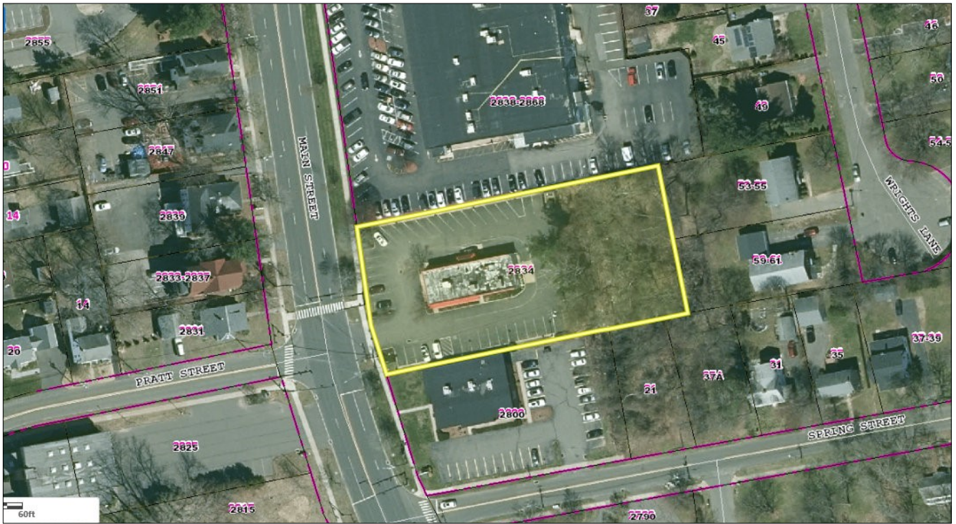
Aerial view of 2855 Main Street looking west
