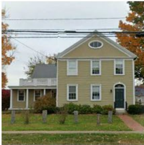
SOUTH OF PROJECT SITE
