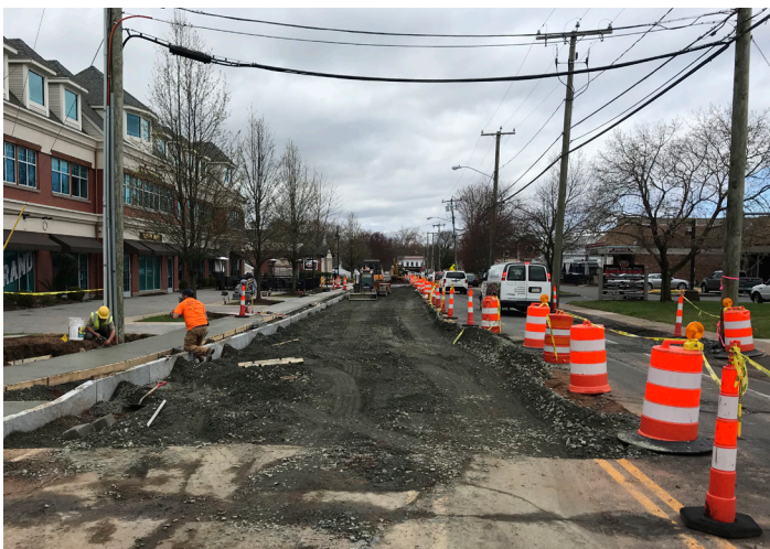
Hebron Avenue Pavement Rehabilitation
