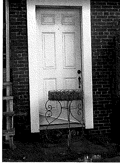
Door on Patio to Office
