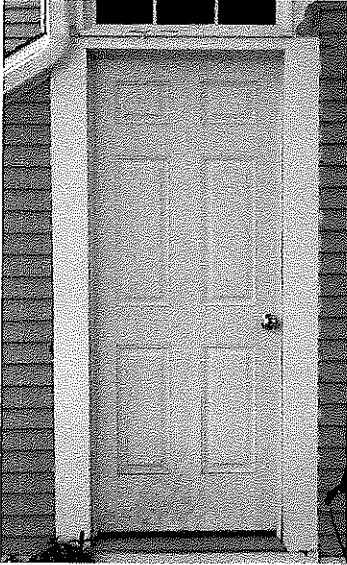
Door on Patio to Kitchen
