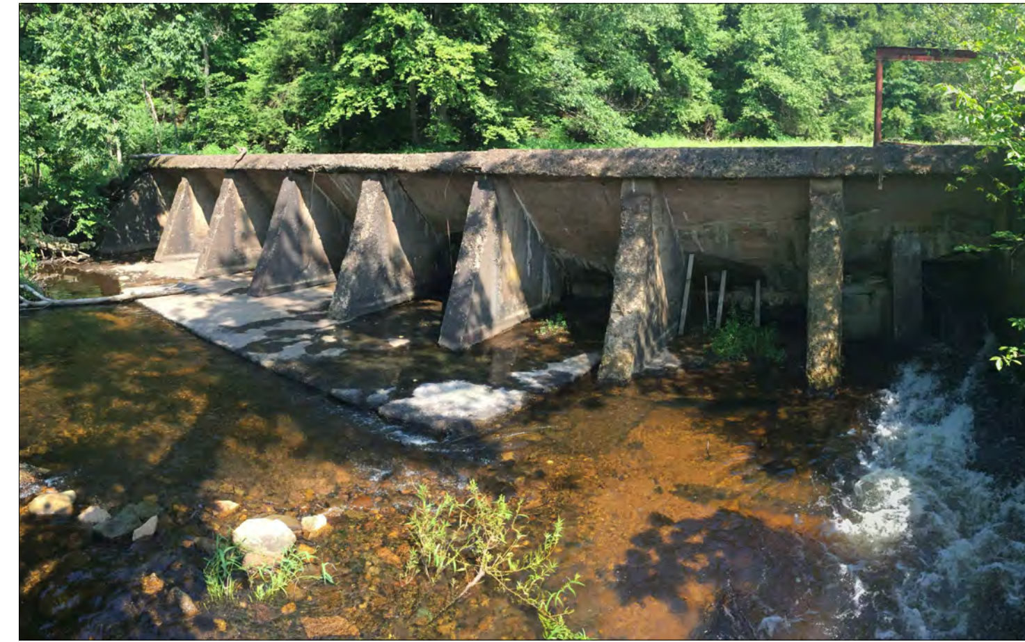
B ORTHOGONAL VIEW OF AMBURSEN SPILLWAY PHOTOGRAPH
