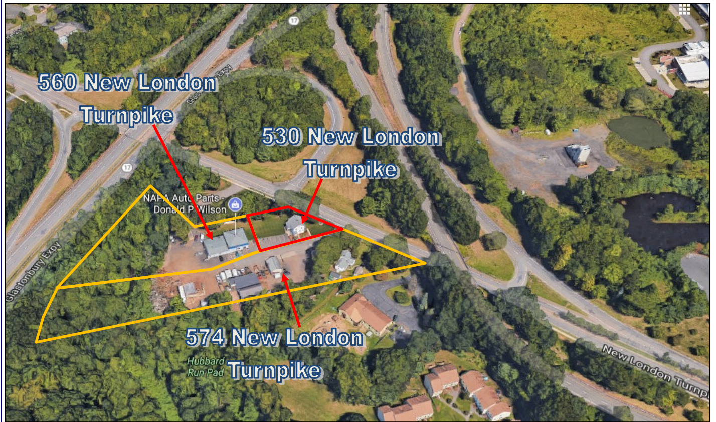
Aerial view of 530 New London Turnpike looking north
