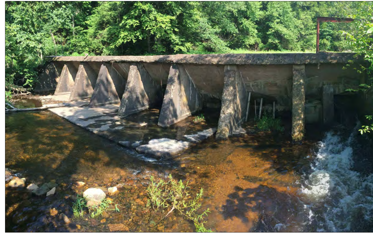
B ORTHOGONAL VIEW OF AMBURSEN SPILLWAY PHOTOGRAPH
