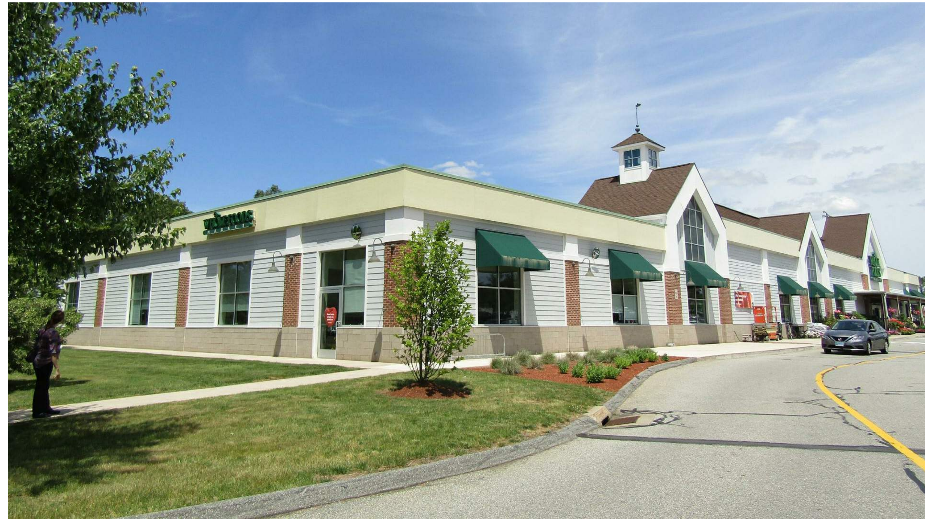
3 WEST FACADE - EXISTING 1/2" = 1'-0"
