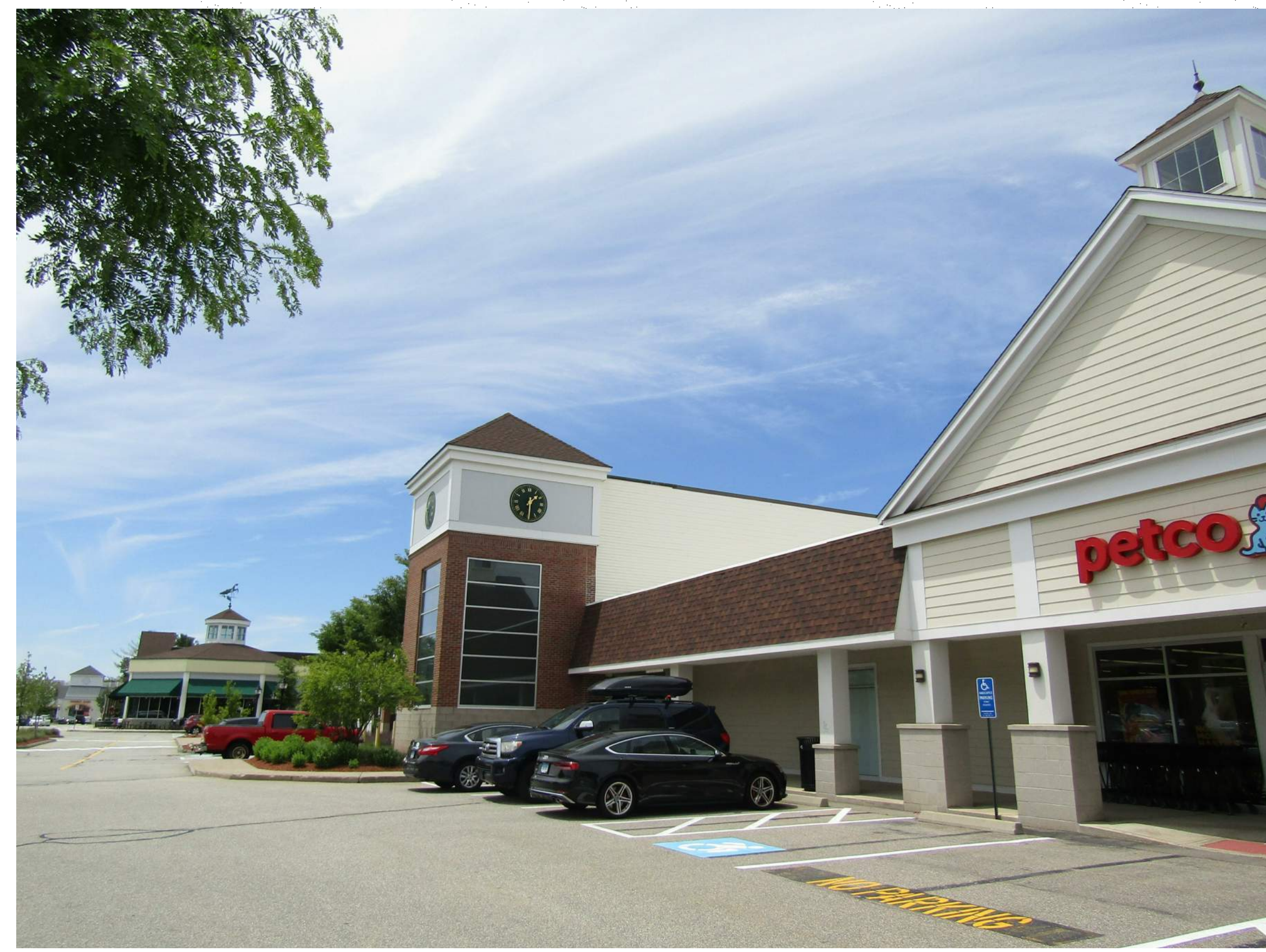
7 LOBBY TOWER - EXISTING IMAGE 1/2" = 1'-0"
