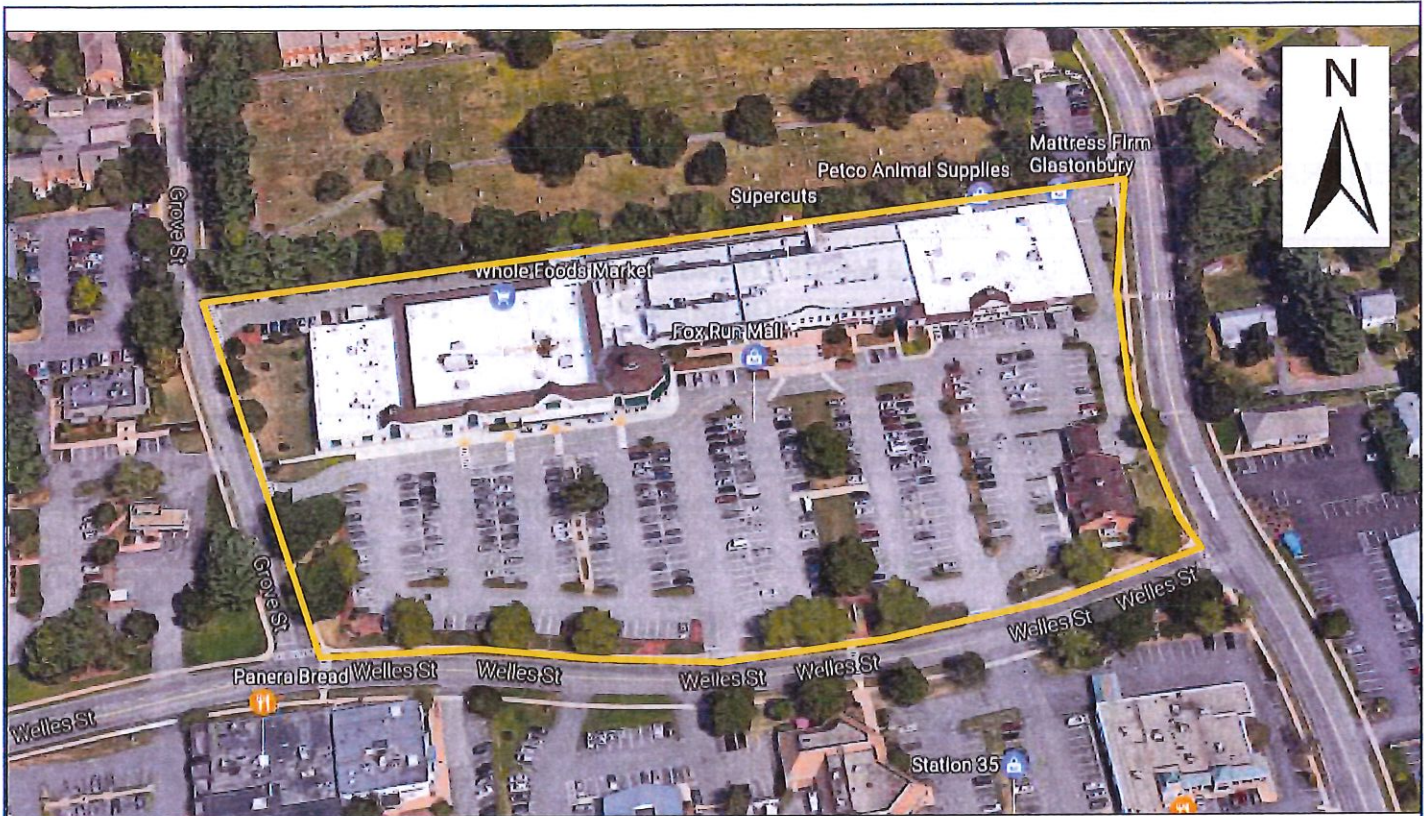
Aerial view of 55 Welles Street looking north
