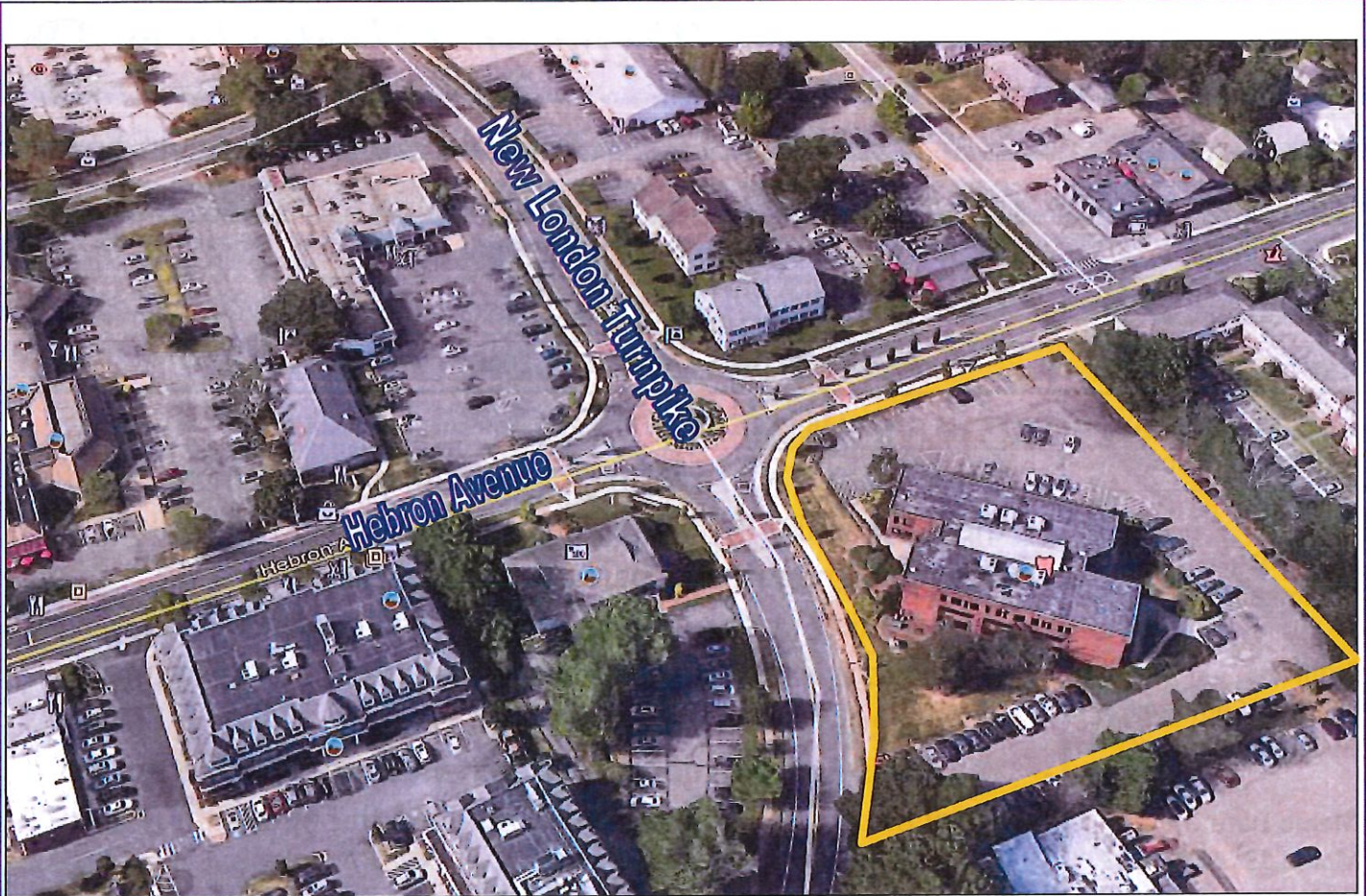
View of 131 New London Turnpike looking north
