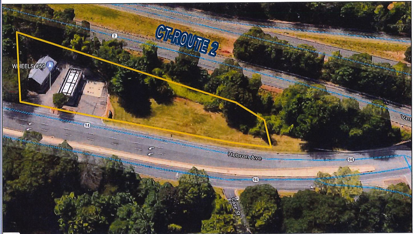
Aerial view of 592 Hebron Avenue looking west
